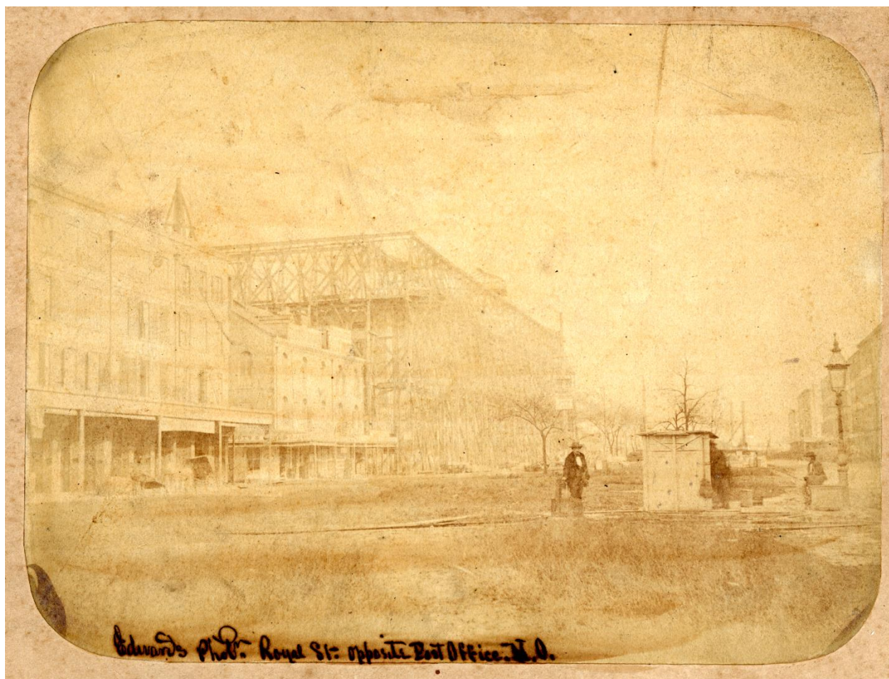
Canal Street, New Orleans, LA. Undated. Showing early construction of United States Custom House. J.D. Edwards, photographer.
