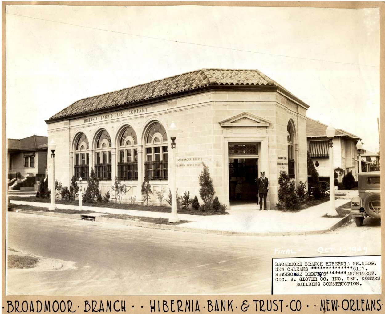
Hibernia Bank and Trust Company, Broadmoor Branch, Broad Street and Washington Avenue, New Orleans, LA. 1929. Rathbone DeBuys, architect. Photographer unidentified.
